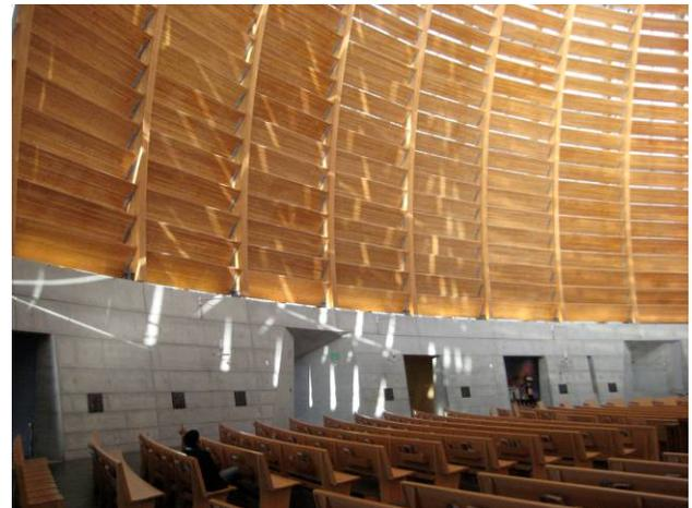
**FIG. 4 INTERIOR VIEW OF CONCRETE RING AND WOODEN VAULT IN DOUGLAS FIR**
